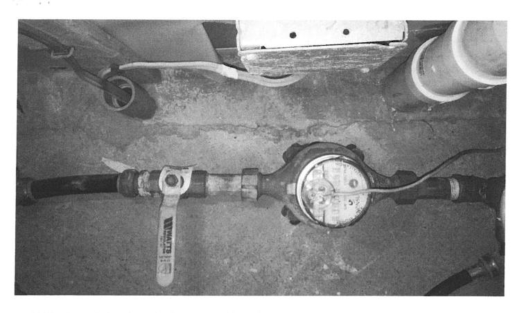
This is a picture of where the crack in the meter is and this is where water was leaking at no more than 2-3 gallons per hour.
