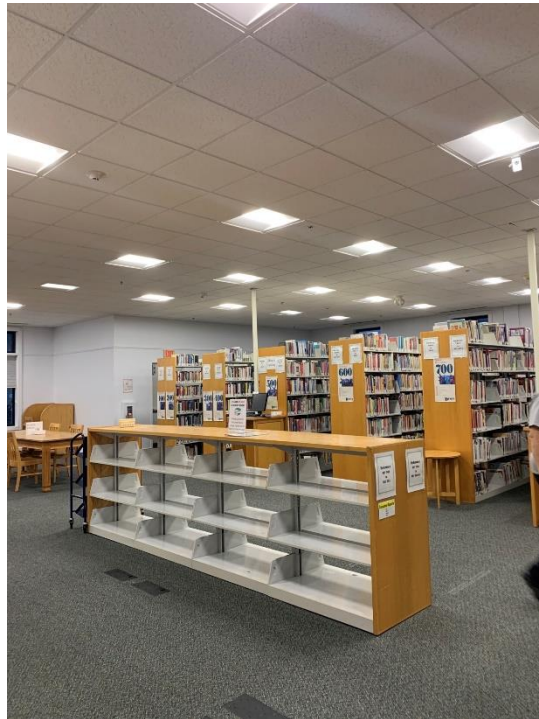
Library LED lighting upgrades
