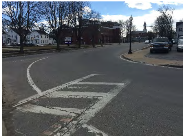
Figure 2-1: Crosswalk #2 with no signage and worn striping
