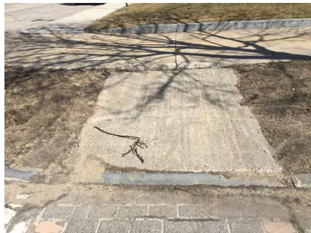
Figure 2-3: Non-ADA Compliant Curb Ramp with step
