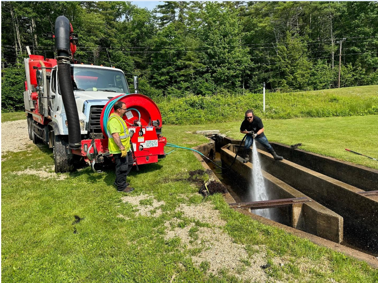
Sluiceway Cleaning 2023
