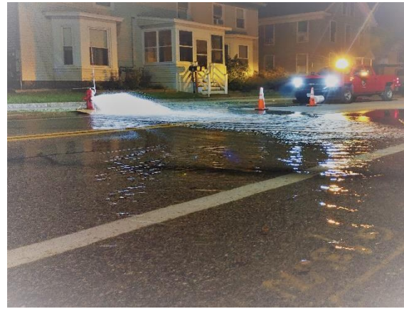
Water main flushing on Portland Avenue
