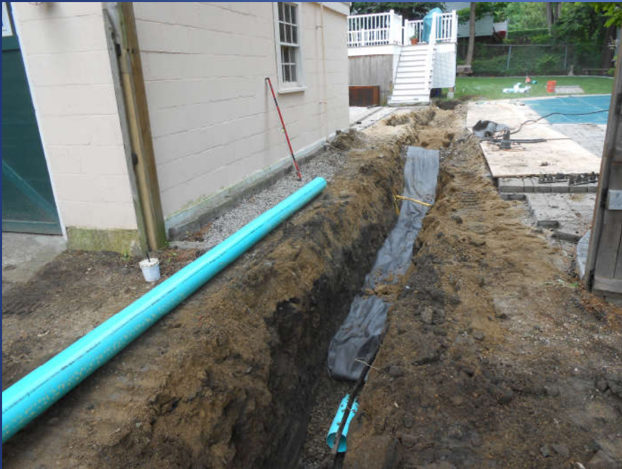
Sewer construction beneath paver patio adjacent to pool
