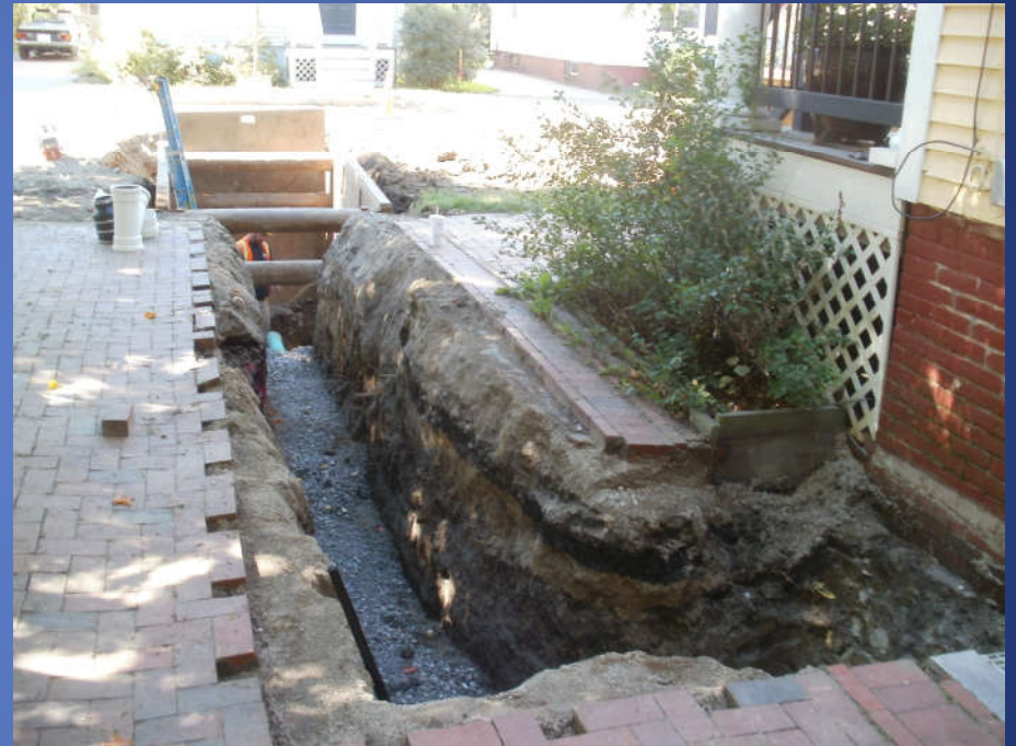
Sewer service construction beneath brick driveway
