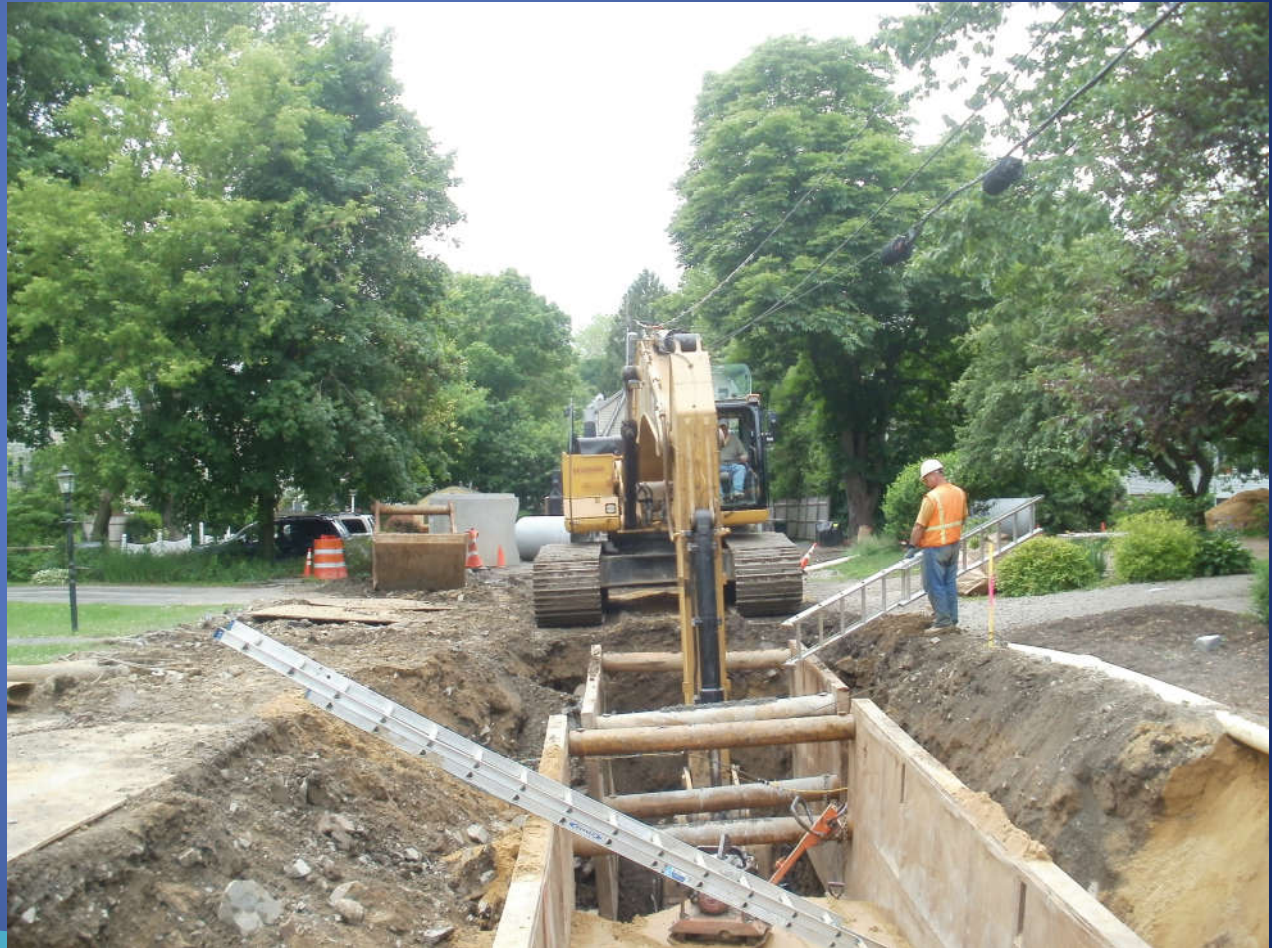
Typical Sewer Main Installation
