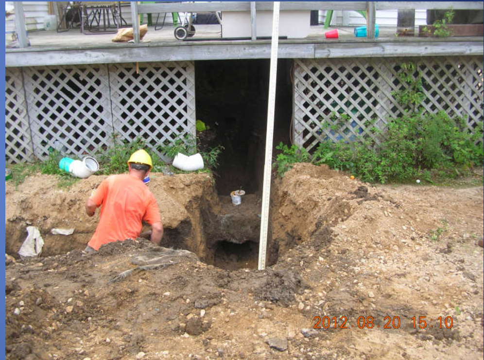
Sewer service installation below existing deck
