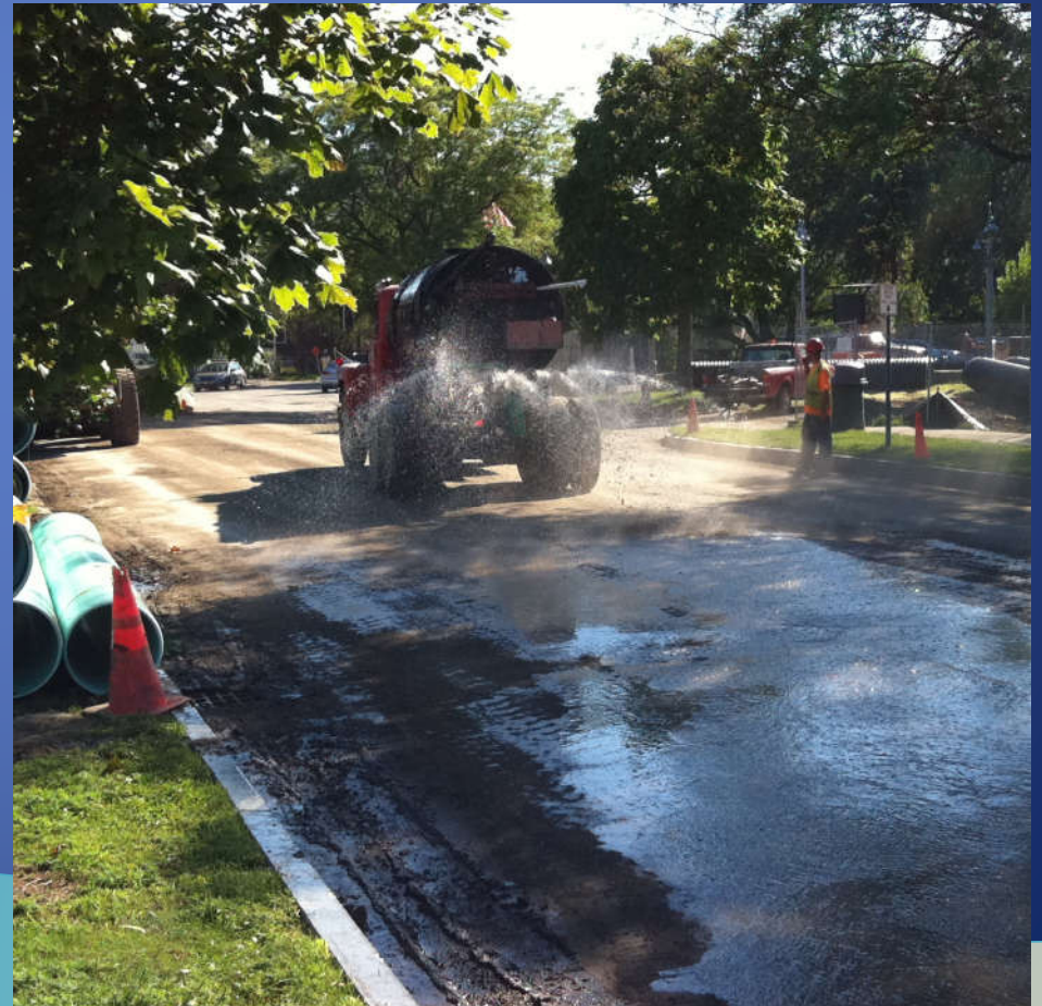
Water truck for dust control
