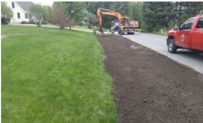
Highway Dept. filling & loaming Tessier Drive ditch line
