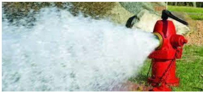
Hydrant Flushing
