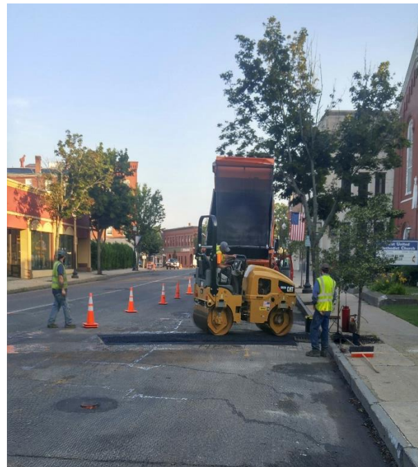
Highway Division repairing a drain line on So. Main Street
