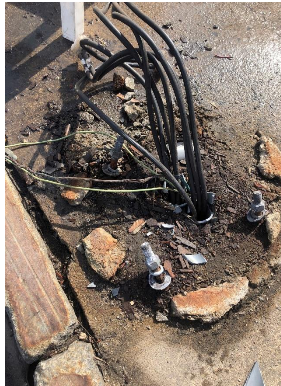
Repaired wiring and mounting and hardware replaced fixture on North Main Street
