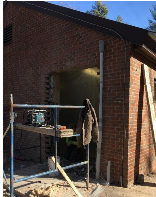
Demolition for the new chemical feed room door at the low lift pump station
