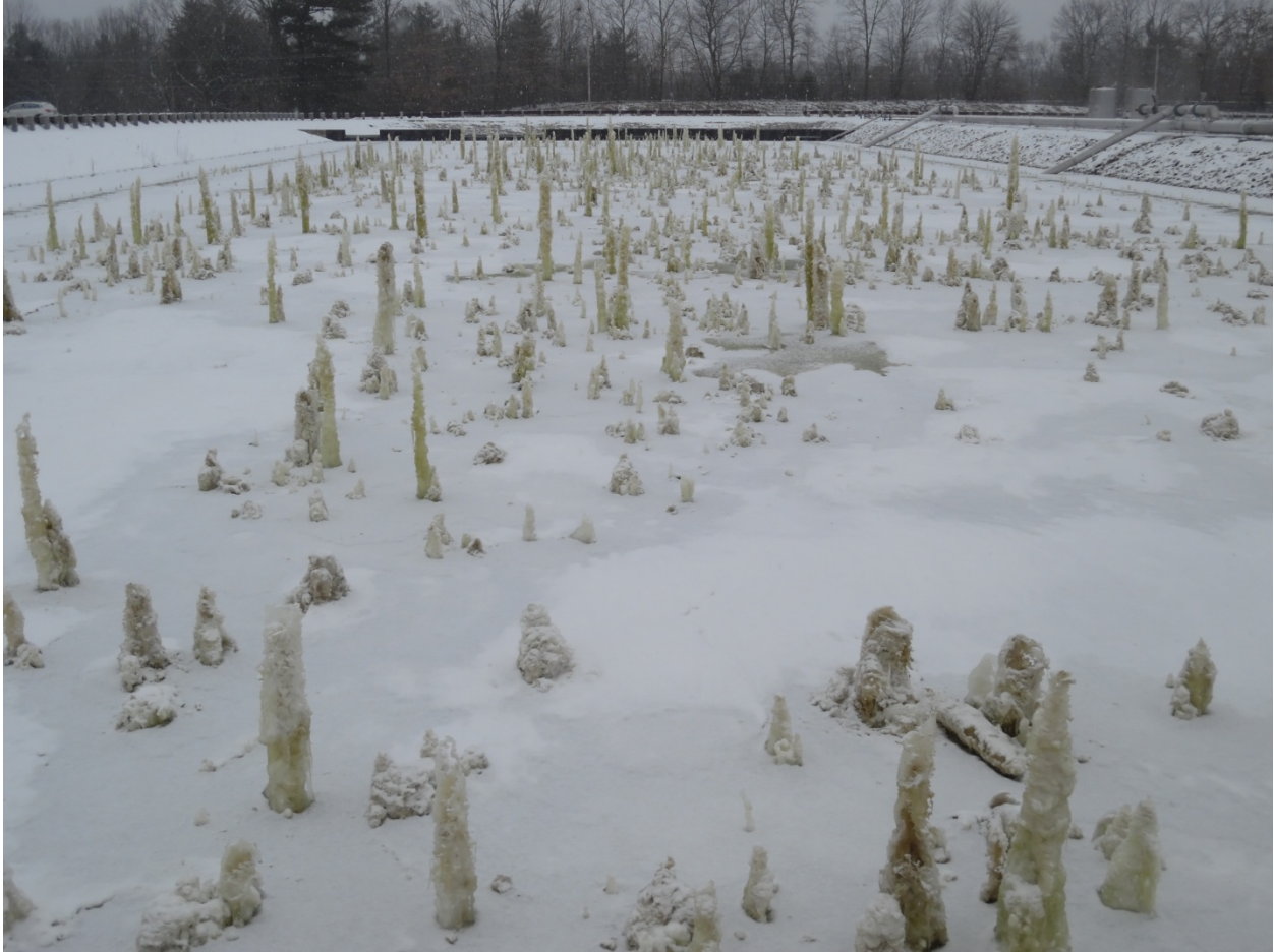
Stalagmites that have formed on WWTP's off-line aeration basin
