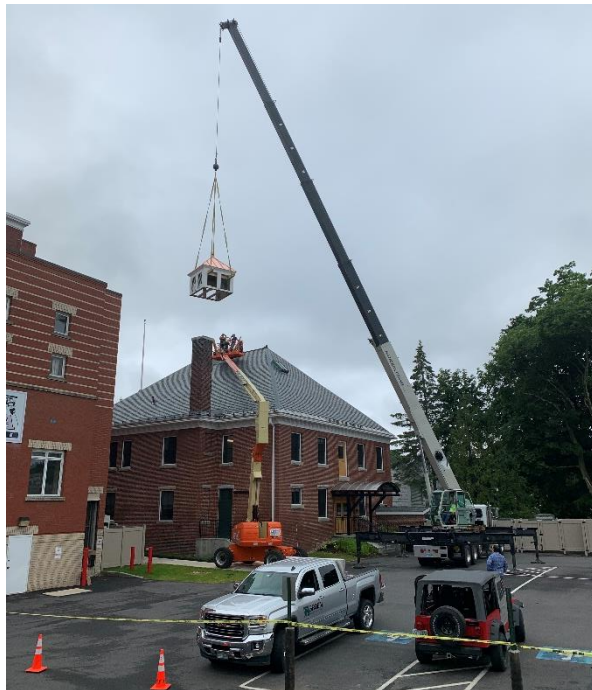
Reinstalling the Cupola on the Annex
