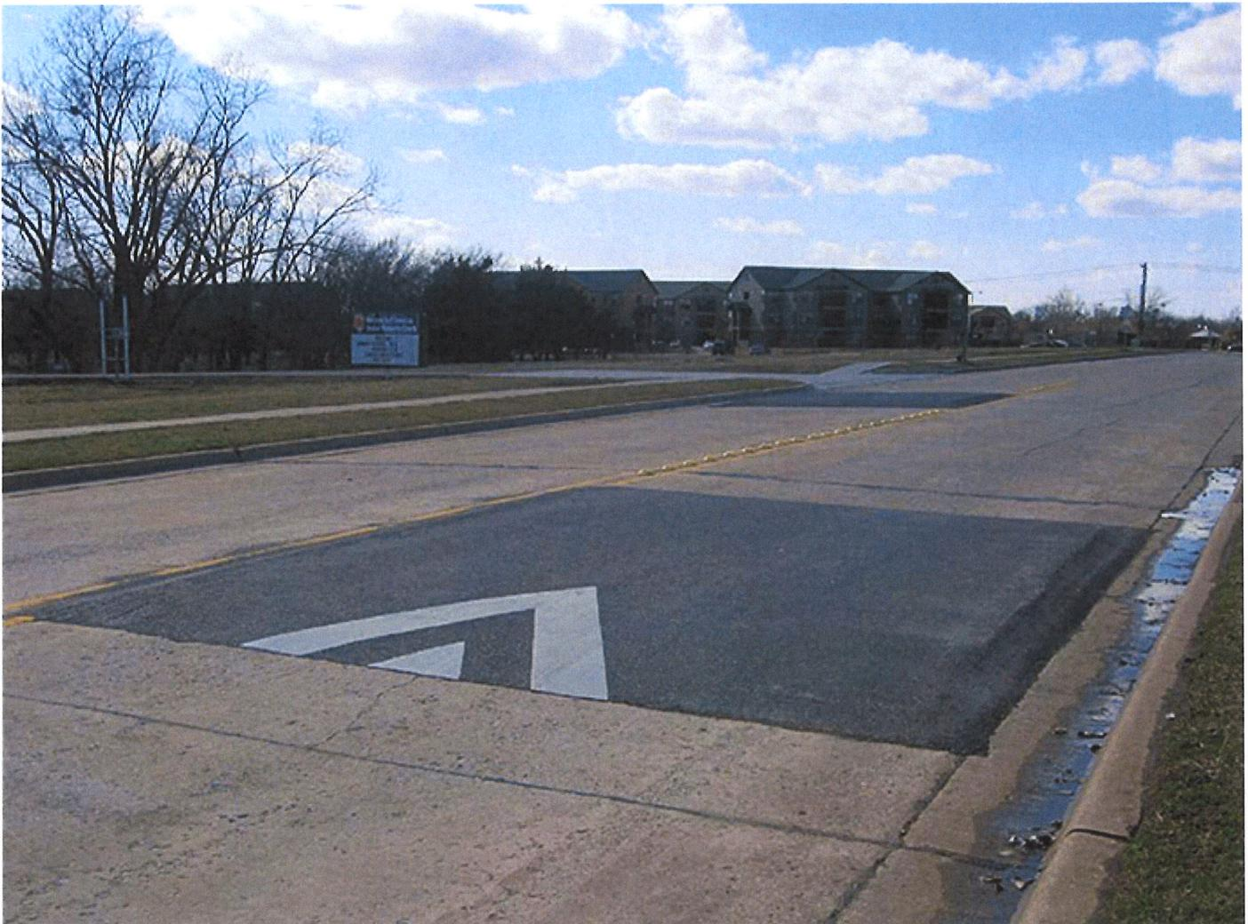
**Figure 5.2. Offset Speed Table with Raised Markers Between the Offset**
