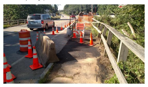
As the project got underway, we learned that NH DOT would require a significantly upgraded guardrail system that was designed to restrain a vehicle from tumbling into the Cocheco River. The guardrail system had to withstand a vehicle impact and also be tall enough to serve as a handrail for people approaching the pedestrian bridge. Additionally, a section of the guardrail would have to be affixed to the bridge abutments. A sample photo of possible alternative is attached.
