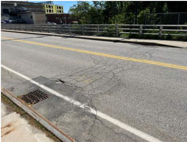
*Pavement Cracking at South Approach*
