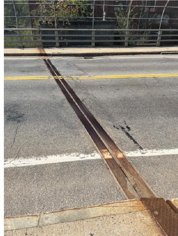
*Expansion Joint Filled with Debris*
