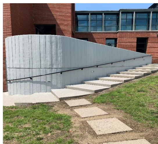
Dry locking of library retaining wall
