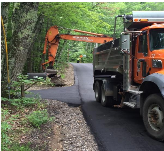
Repaired washout on Four Rod Road
