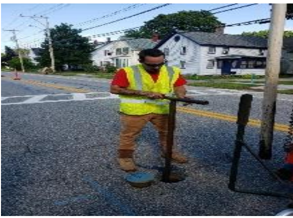
Cleaning mainline gate valves
