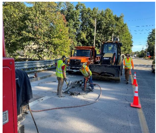
A crew repairs a failing sewer manhole on Route 125
