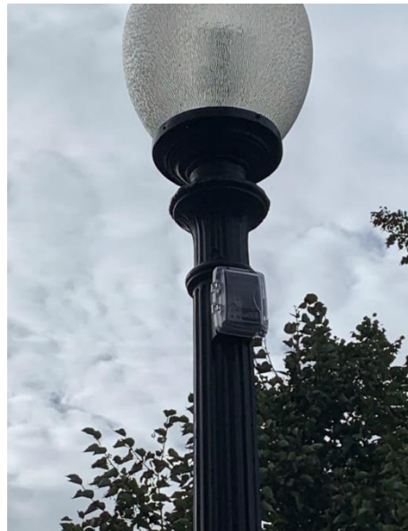
New circuits, wiring and outlets at the Commons
