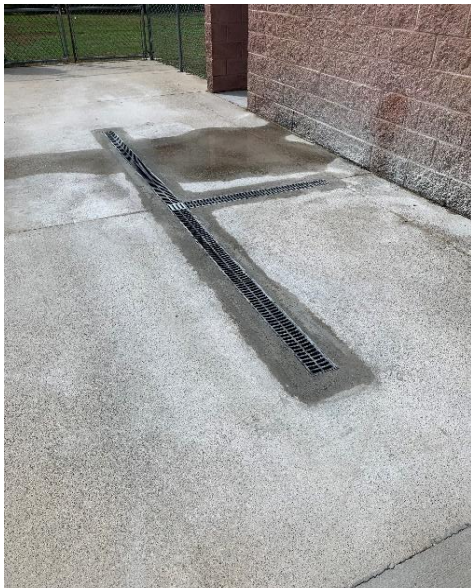
Installed new floor drain in Hanson Pines pool showers
