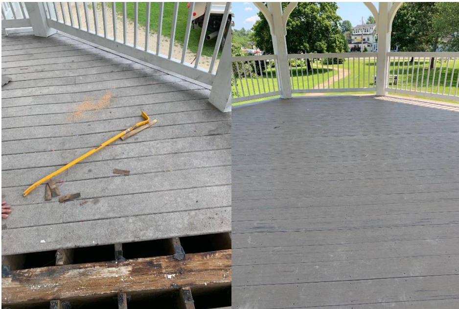
Installation of Decking on Bandstand at Rochester Common
