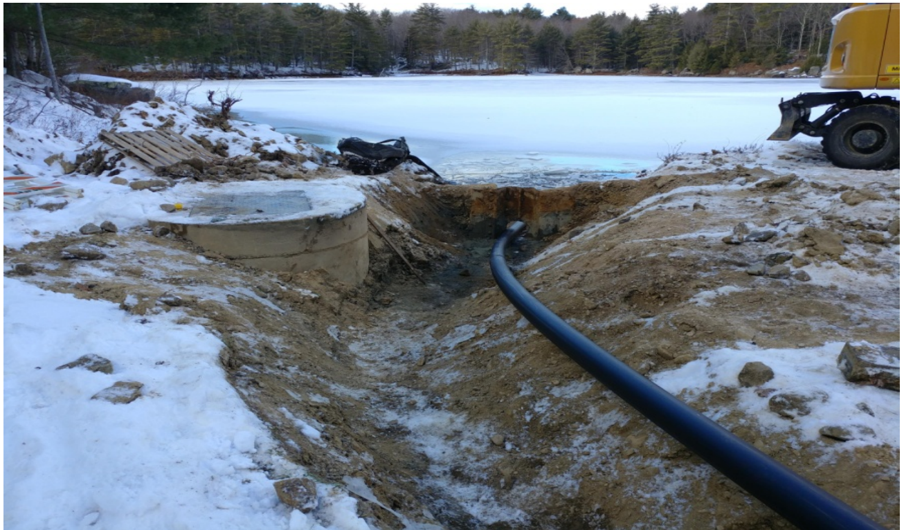
New air sparge/scour line to the intake
